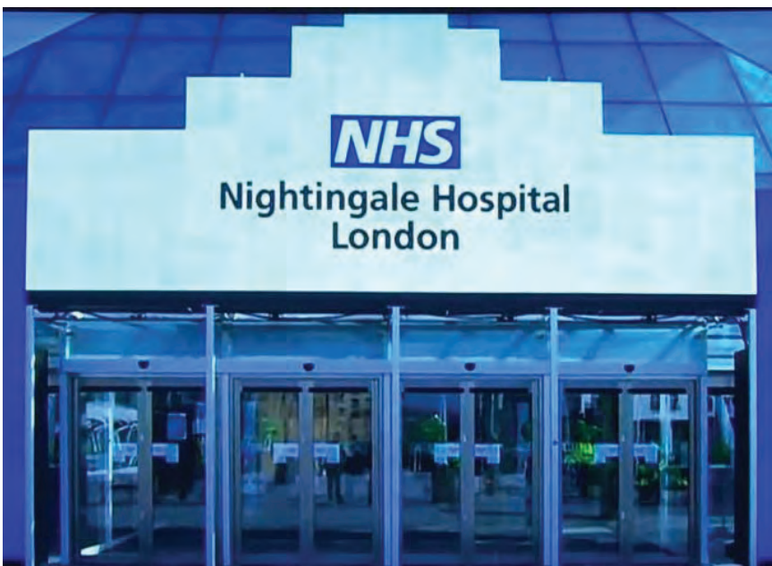
The finished Nightingale Hospital.
