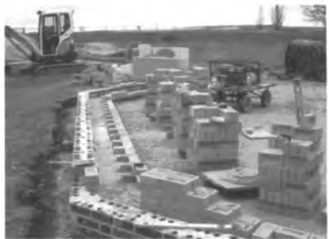
Brickwork for the bench seating.
