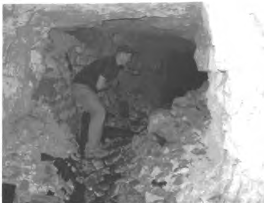
OC HQ Coy Potholing in a minor fort communication tunnel.
