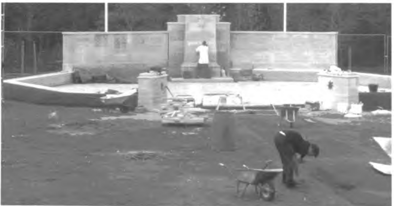
Landscaping and laying the path.
