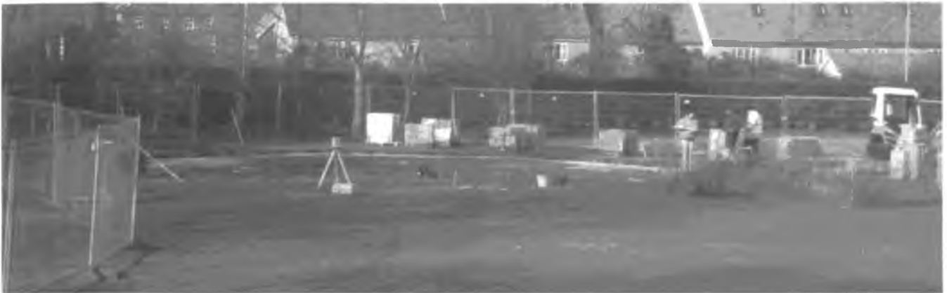
The site is cleared.
