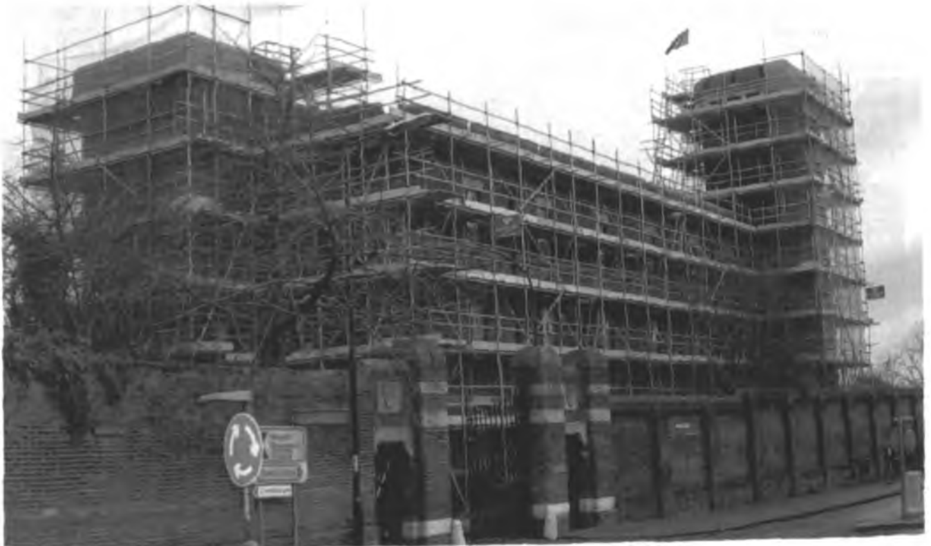
The Keep, shrouded in scaffolding.
