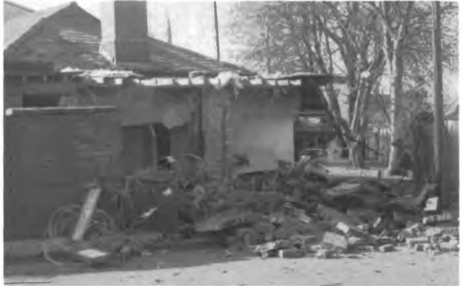
Damage to the old guardroom.
