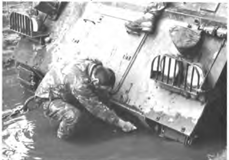
Working conditions on Soltau
