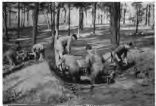
Digging in the Signals Centre during training at Sennelager.
