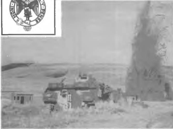
Blowing the bridge — B Coy at Batus.
