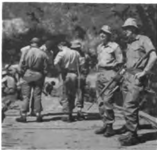
'Pioneers Bridge' . . . Sgts. Lowe and Blower.
